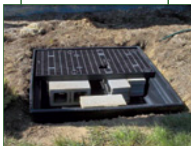
C. Add Cinder block and pump assembly.
